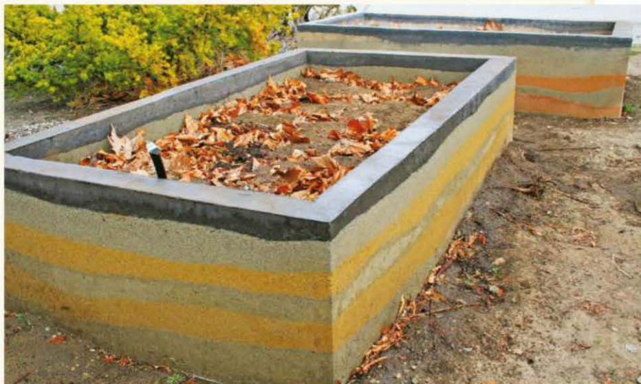
Rammed earth garden beds absorb heat during the day and release it at night.
