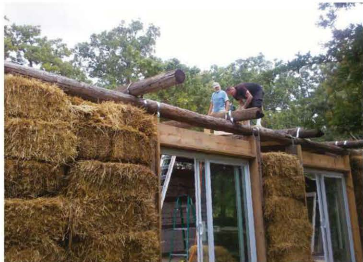
Though drought made straw scarce in Texas, the Poupores sourced enough to build their straw bale home. Reclaimed telephone poles support the roof.
