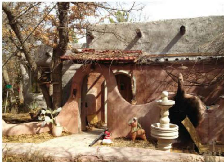
Though drought made straw scarce in Texas, the Poupores sourced enough to build their straw bale home. Reclaimed telephone poles support the roof.
